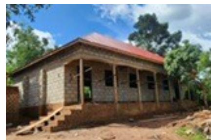
Completed Dormitory, January 2025
